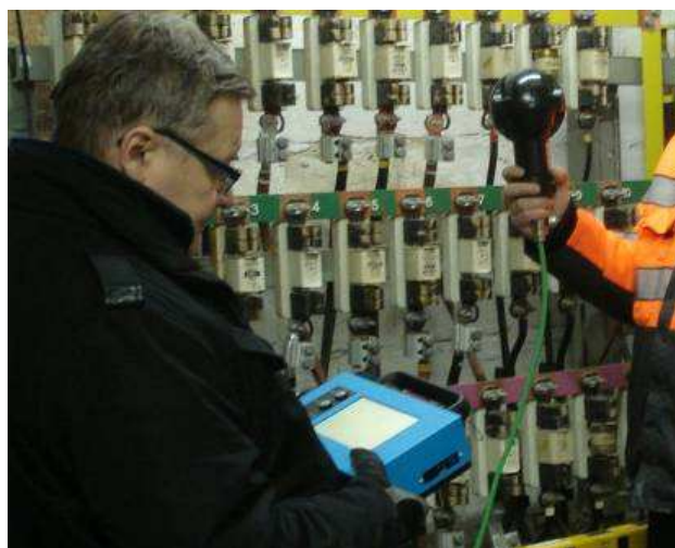
Figure 1: Measurement Place A, near fuse panel.
